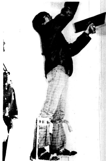
TALL MAN IS Jim Bucher as he dons a pair of special stilts to plaster ceiling in building trades class. Boys from Akron and Mentone high schools have combined their talents this year under the direction of Charles Fellers. Far left, a licensed vocational teacher, in building a new house in Mentone, the seventh house built by TVSC students. Superintendent of TVSC schools Robert Forbes said he thinks the program is very successful, basing his conclusion on follow-up reports he receives. In the past, the classes have been conducted on a full-day basis but were offered half-time this year. The boys seemingly have adapted to the shorter schedule well and report having learned many new skills. More pictures elsewhere in the NEWS.
