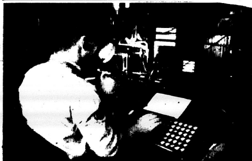
Bill Horn, lino-type operator, is shown operating the Linotype which casts the lines of type used in composing the news stories and advertisements. An Intertype assists in the linecasting and is also operated by Mr. Horn.
