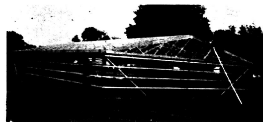
YOUTH LEAGUE PAVILION takes shape at Mentone. The 40' x 64' building that is being built at a cost of $5500 is taking shape on the Youth League lot. It will be covered with aluminum panels and will have suspended ceilings and complete restroom facilities. Jerry Secrist, president of the League, says it is hoped the building can be in operation by Aug. 1 and that it will be available to any groups wishing to use it. In addition to the new pavilion, work has begun on a tennis court.
