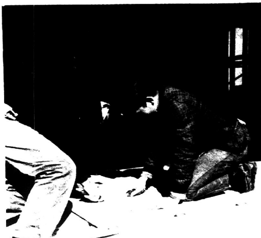
IF AT FIRST IT DOESN'T FIT you re-cut it, these Mentone boys have learned. Richard Morrison and Cam Rathbun shown retrimming the dry-wall panel.
