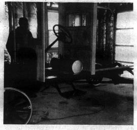
MIDWAY through the preservation process, truck looked like this as Miller built a frame cab called a "C cab" because it looks like an inverted C.
