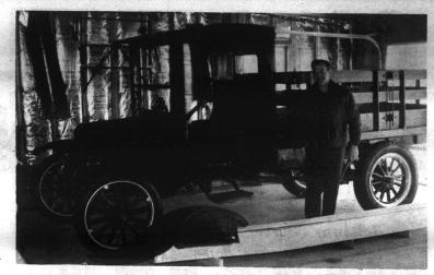
ALMOST DONE, Jack Miller, hammer in hand, has only a fender to install and the preservation of his 1919 truck will be complete. Note the authentic tires, the rebuilt bed and stake sides and the light.
