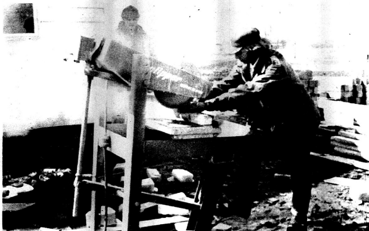
WATCH MY DUST could be what Randy Brown is saying as he cuts a piece of limestone for trim in front of the house TVSC building trades students are erecting in Mentone. John Meade watches.
