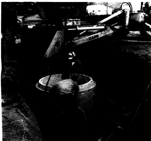
THE MANHOLE IS seated on a base and the joints are then sealed.
