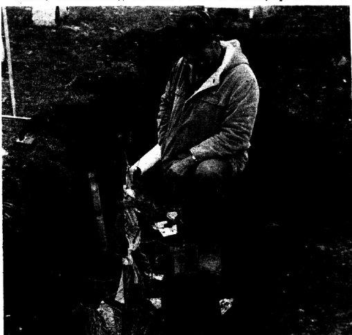
NORMAN BENSON, an employee of General Telephone Company, pauses as he reconstructs a telephone cable that was accidentally snapped by workers installing Akron's new sewage system.
