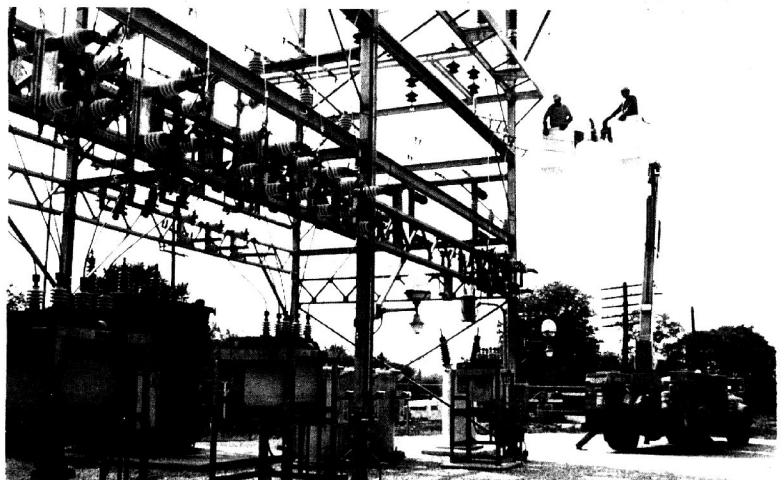
MENTONE POWER IMPROVEMENT - Roy Hauth (left) and Jack Culbertson, Northern Indiana Public Service Company linemen, make some final adjustments on the utility's Mentone Substation. The station was recently modified and expanded to provide two 69,000-volt supply lines with automatic change-over, two 69,000 to 12,500-volt power transformers for additional flexibility and three 12,500-volt distribution circuits with automatic reclosing. "Completion of this program will provide both the town and surrounding rural area with a more reliable source of electric service," said Charles A. Heim, NIPSCO Warsaw district manager.
