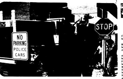
...And then Rochester Street (SR 14) from SR 19 to SR 114 by Cooksey's Freezer Fresh was literally "pulverized." Contractors used a pulverizer to remove about four inches of pavement. New asphait will be laid this week.
