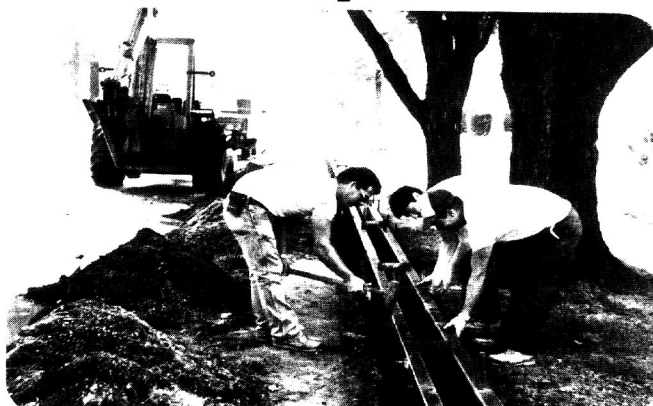
The curbing project continues to progress in Mentone despite the recent showers. Gremmen for Secrist Builders are shown installing the curbing forms on Tucker Street before the cement was poured. (NEWS Photo)
