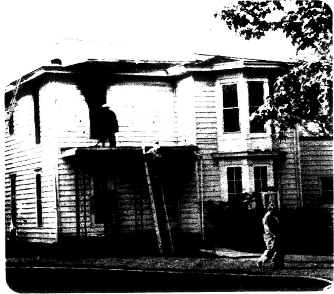
Fire officials have not yet determined the cause of the fire that damaged the home of Dave Croushore at Orchard and West Streets, Akron, on September 8. The fire was contained to the upstairs area with damage believed to be between $4,000 and $5,000. (News Photo)
