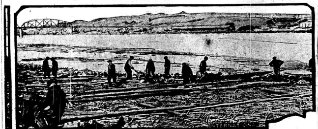
Workers near Mandan, N. D., rip-rapping the banks of the Missouri river as protection against the expected spring freshets. The work consists of laying rock on willow mat and sinking it in the river. Liberty Memorial bridge is shown in the background.
