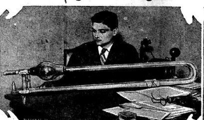
A new beacon light which is reported to be the last thing in beacons as an aid to both aerial and water navigation has recently been invented by a former Cornell student, R. R. Macbeth of Long Island City. The light is of hairpin shape, double backed, each unit producing 10,000 candle power.
