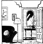
CRACKED WALLS—Often caused by uneven settling of footings and foundation. Skimping on footings in either size or concrete mix is poor economy.
