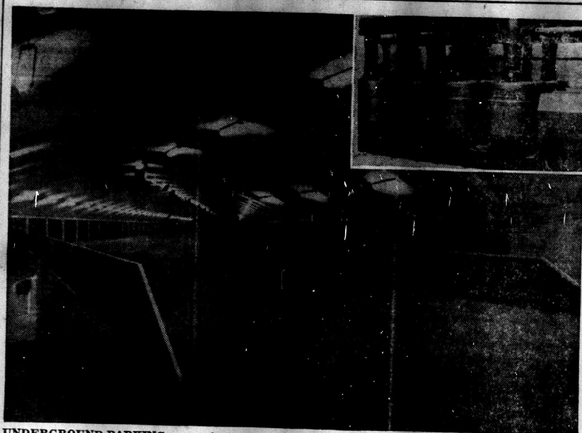
UNDERGROUND PARKING garage in Stockholm, Sweden, showing two levels in this vast dual-purpose civil defense shelter which can accommodate 10,000 persons. The garage, a key unit in the largest underground shelter program in the world to-
