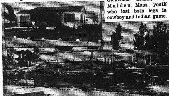
A NEW HOME IN 5 DAYS. Miami, Fla.—Five days after erection starts, a new Tec-built house is ready for occupancy. Pre-fabricated sections are loaded into two Fruehauf truck-trailers for speedy delivery to the jobsite
