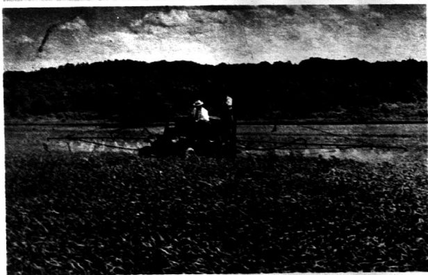
Ingenuity! A jeep (or truck), a 42 foot boom with spray nozzles set 18 inches apart, three discarded oil barrels filled with recommended weed killer, and any farmer can rid his fields of thistles and wild mustard. County Agent E. M. Skaliskey of Washington County, Wisconsin, is shown on the jeep fender.
